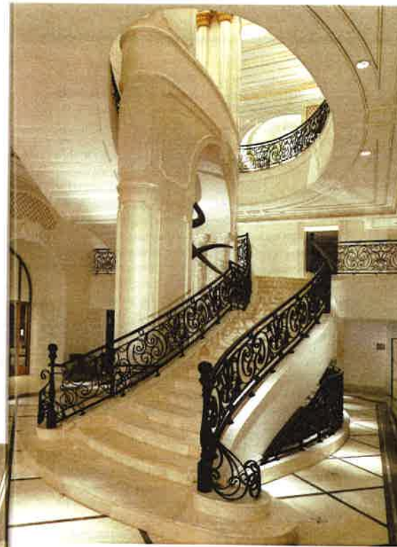
The entrance lobby features a grand staircase that is clad in marble and has an intricate ironwork railing. The central, decorative arch conceals the concrete column from which portions of the stair cantilever 1.5 m.
